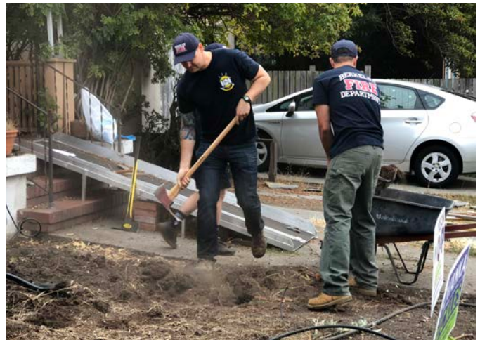
TWO BERKELEY FIREFIGHTERS DIG IN JULIA'S YARD
